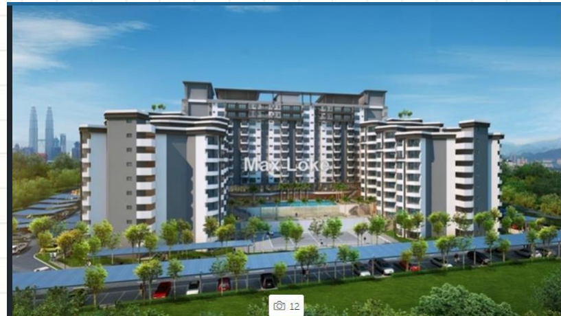
1 Harmonis Condominium @ Gombak – AGA Development Sdn Bhd
