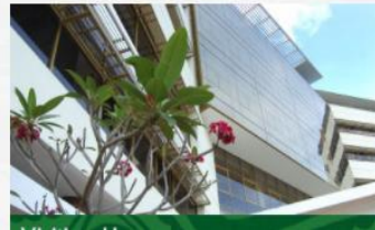
Regeneration Health Rehabilitation Centre, Petaling Jaya
