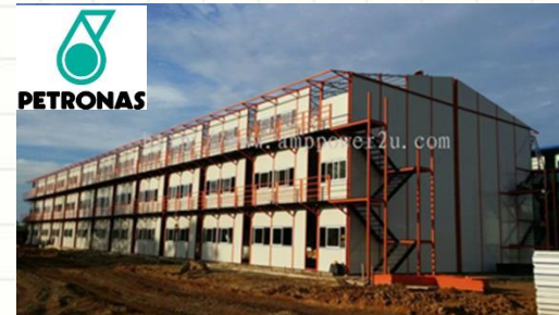
Petronas Rapid Temporary Executive Village, Pengerang, Johor - Petronas
