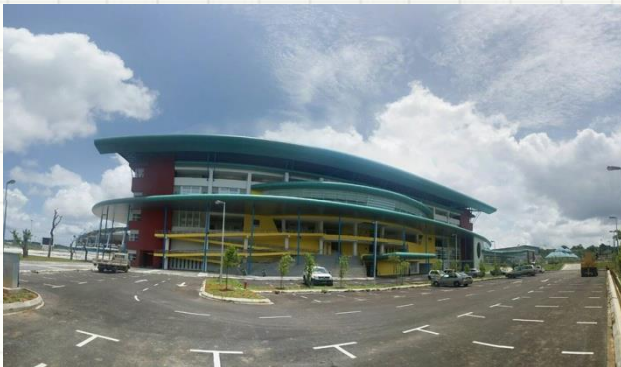
Sarawak Sports Complex, Aquatic Centre Petra Jaya, Sarawak.
