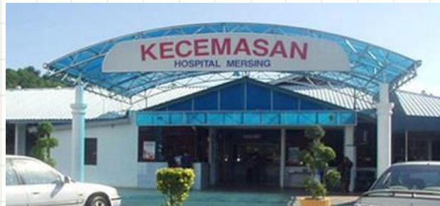
Hospital Mersing, Perak
