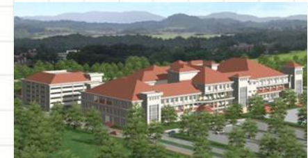
Taiping Hospital, Perak
