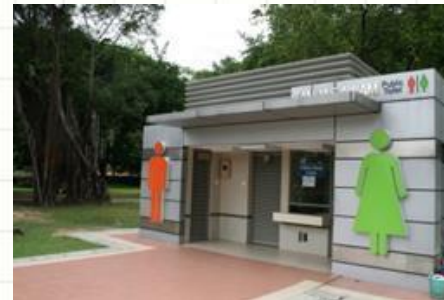
Kuala Lumpur City Hall's Public Toilet - Automatic Street Toilet, Fully Automated & Anti vandalism
