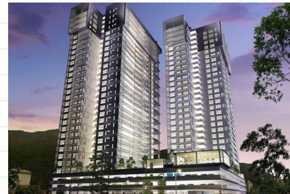
Condominium Berjaya, Bkt. Mertajam, Penang – Five Star Contract Sdn Bhd
