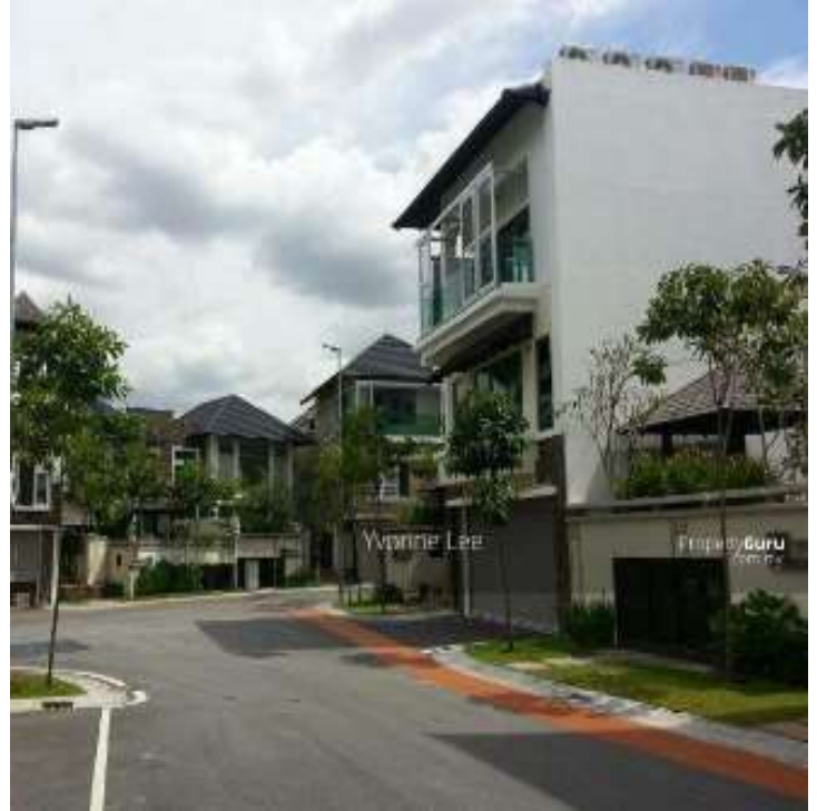
PROJECT : THE VILLA @ SERAI SAUJANA LOCATION : SHAH ALAM (SELANGOR) DEVELOPER : SERAI SAUJANA DEVELOPMENT
